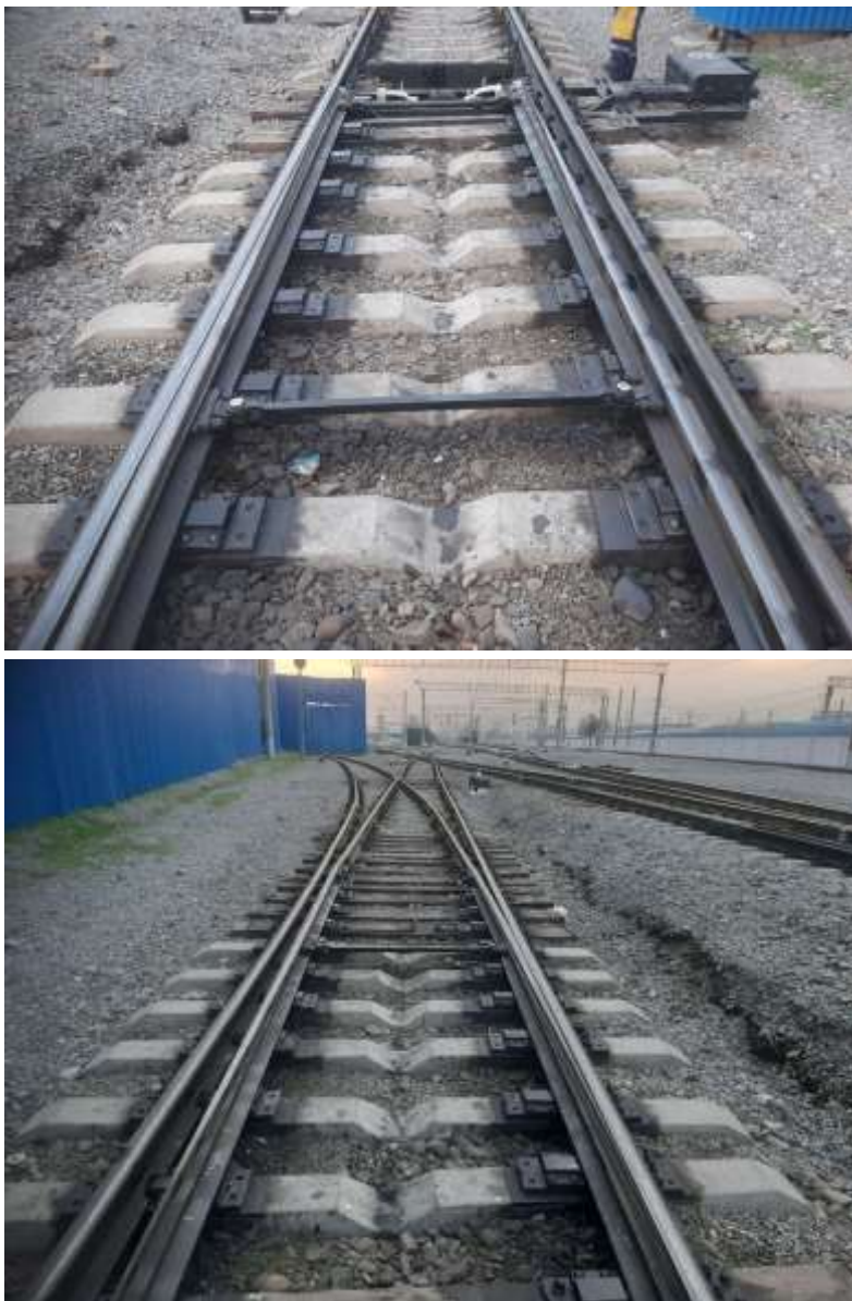
2-rasm. Strelkali o'tkazgich markasi 1/9, Rels R50, 6 ta temir beton bruss.
